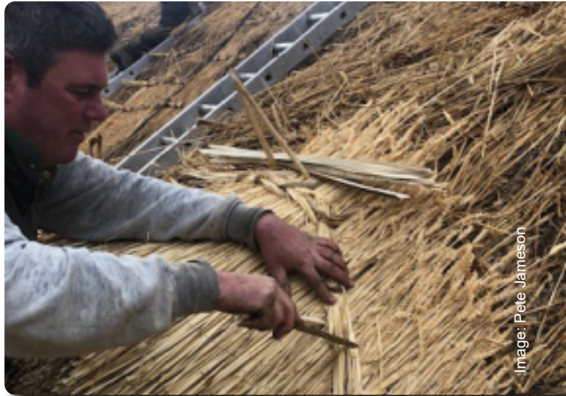
Nigel Turton using Devon spars
