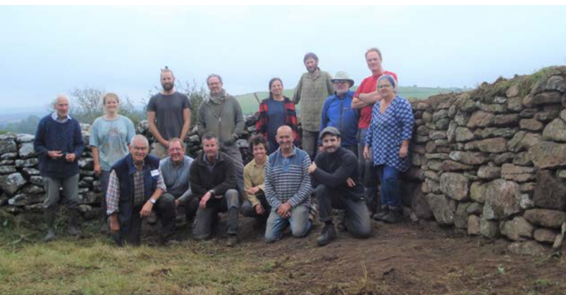
The wall and wallers
